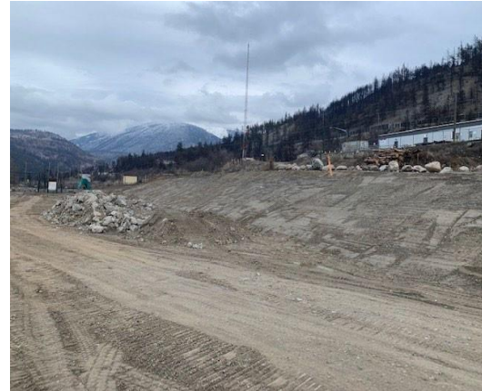
Photo 6 – Concrete Retaining Wall Removed 787 Station St.
