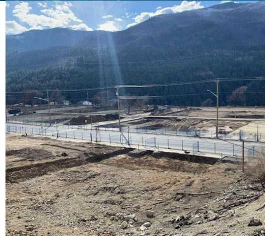
Photo 2 – Zone 5-6 hot spot removal complete
