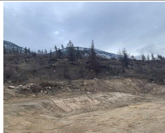
Photo 4 – Zone 3 Hotspot remediation
