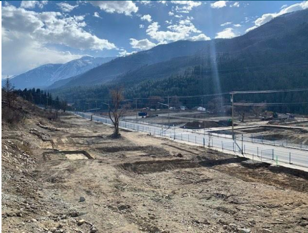
Photo 1 – Zone 1-3 Hotspot Removal
