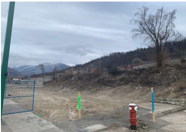
Photo 5 – Concrete Removal and Disposal 421 – 437 Main St.
