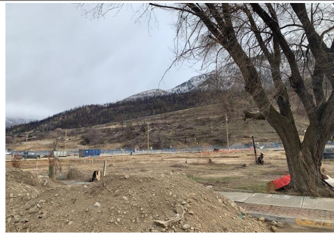
Photo 3 – Zone 2 hotspot remediation.
