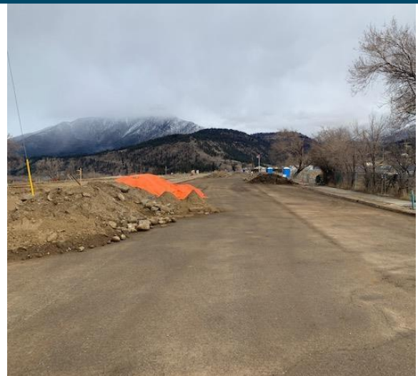
Photo 2 – Zone 1 & Zone 2 hot spot removal complete
