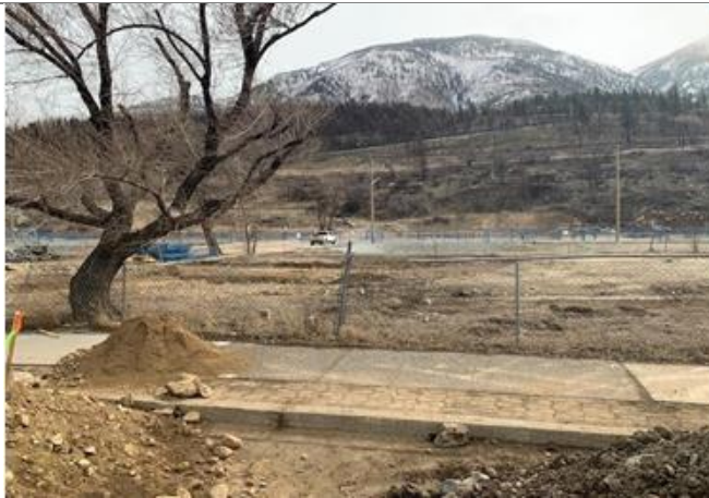
Photo 5 – Zone 3 hotspot remediation
