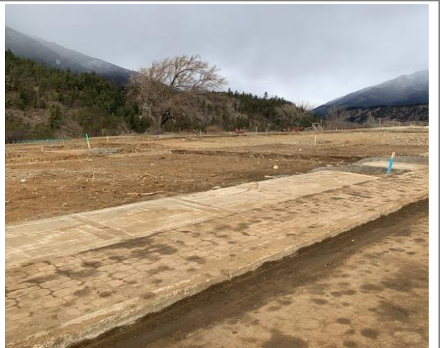
Photo 4 – Zone 3 Hotspot remediation
