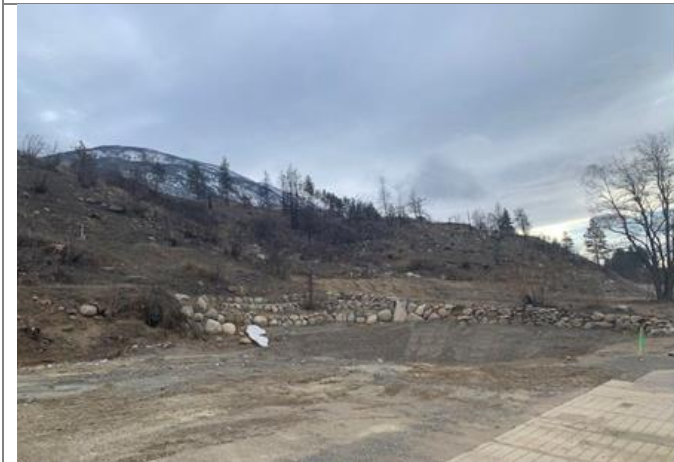
Photo 3 – Concrete Foundation removal and Disposal Lots #125-145 Main Street.
