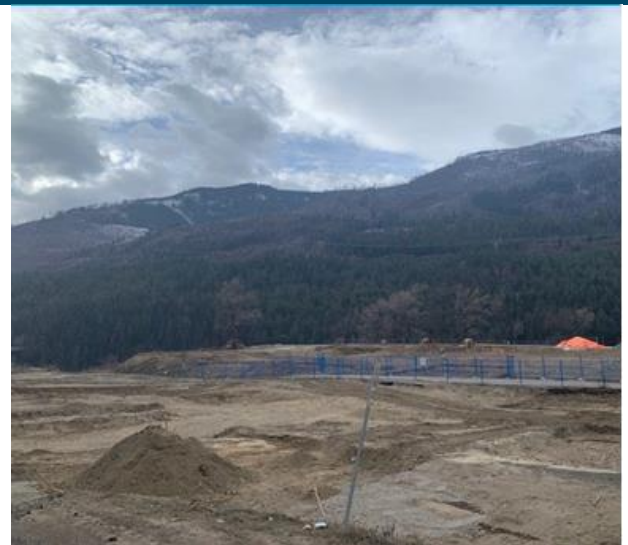
Photo 2 – Zone 1 & 2 hotspot removal complete
