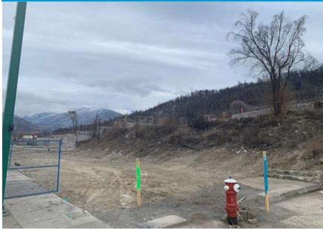
Photo 5 – Concrete Removal and Disposal 421-437 Main Street
