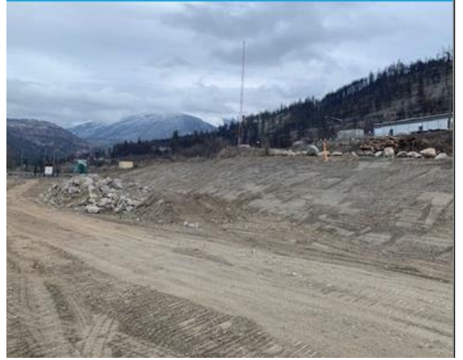
Photo 6 – Concrete Retaining Wall Removed 787 Station Street.
