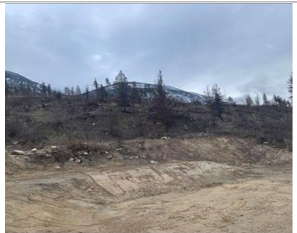
Photo 4 – Concrete Foundation Removed 261 Main Street
