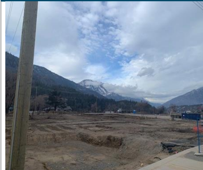
Photo 1 – Zone 1&2 hotspot removal complete
