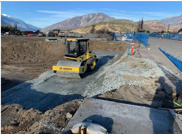
Photo 3 – Retaining wall works in progress west of Highway 12.
