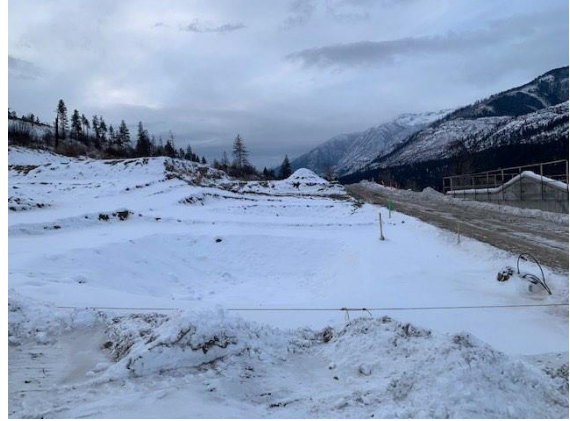
Photo 6 - Zone 3-6 ready for backfill
