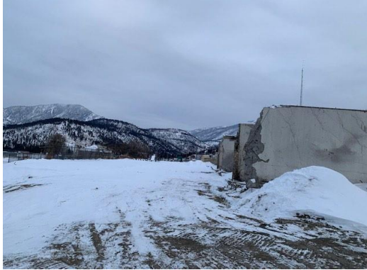
Photo 5 – Retaining walls still pending removal
