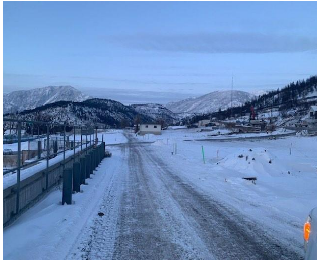
Figure 5 – Site 90% Cleared of contaminated soils.
