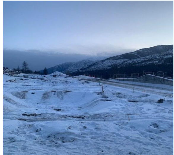
Figure 6 – Sites Prepared for Backfilling
