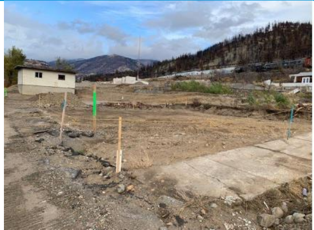
Figure 6 – RCMP site has been cleaned for confirmatory sampling.
