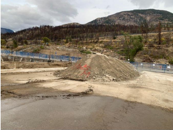
Figure 1 – Haz waste soil mixing has started.
