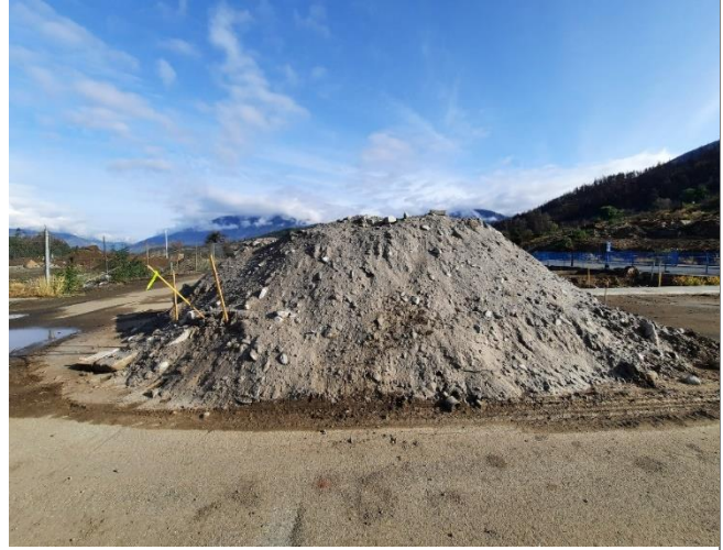
Figure 6 – Portland Cement stabilization of contaminated soils
