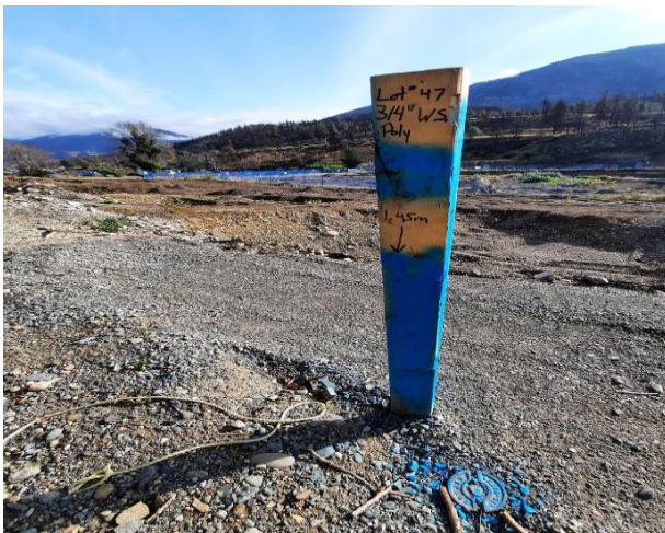
Figure 7 – Capping of Sewer and Water infrastructure
