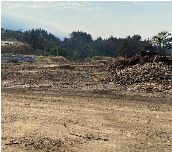
Figure 1 - Zone 1 Remediation Primarily Complete
