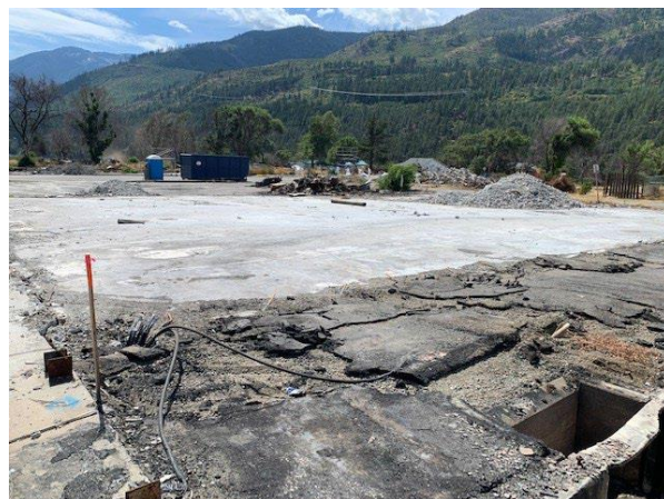
Figure 4 – Grocery Store Demo and Debris Removed
