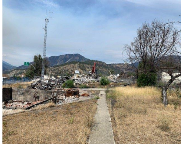
Photo 4 – RCMP Detachment Demo Debris
