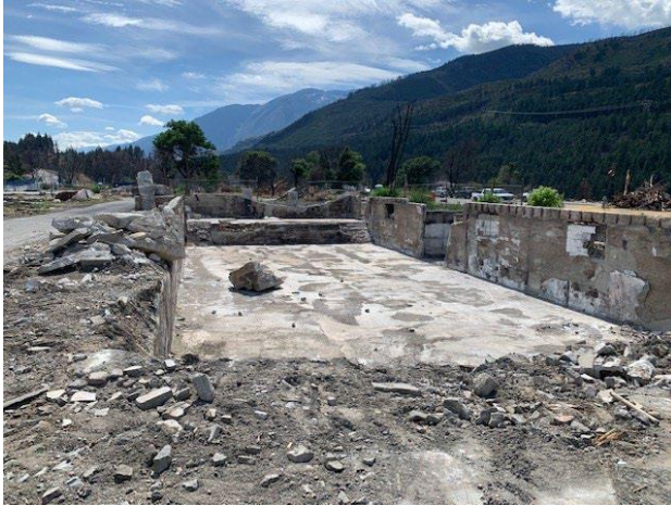
Figure 1 – Lot 141 Debris Removed
