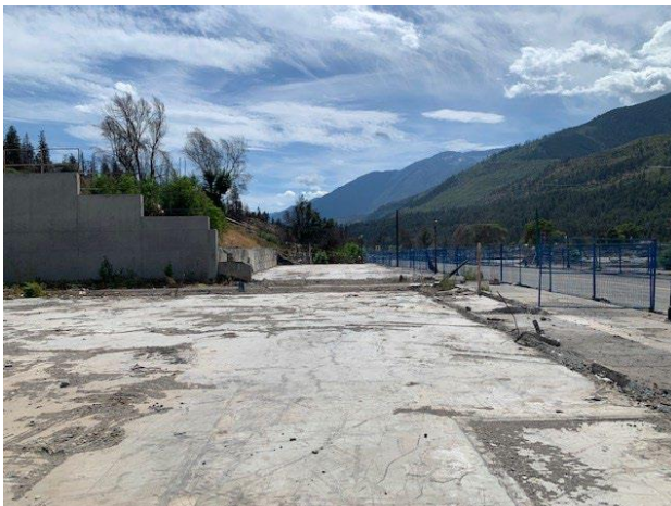
Figure 3 – Scotia Bank Demo and Debris removed
