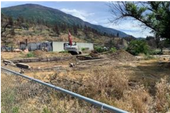
Figure 5 – Lot 665 Zone 6 Debris Removed
