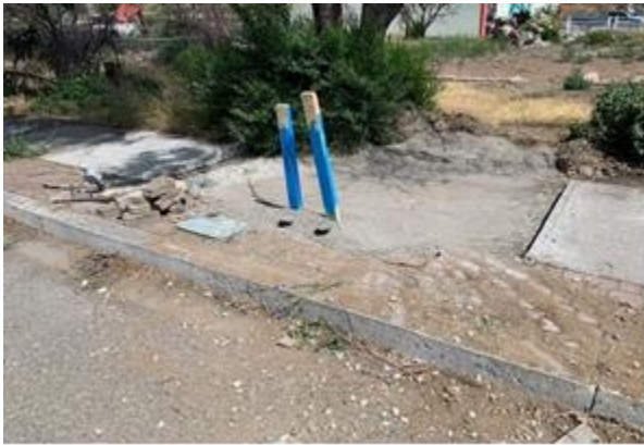
Figure 3 – Utility Cutting and Capping
