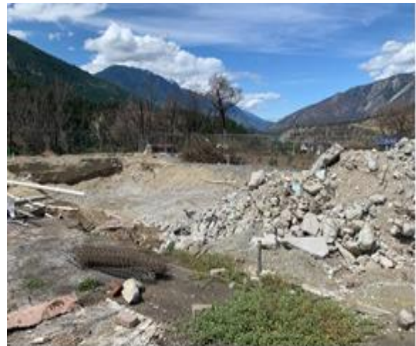
Figure 2 – Pool Demolition Complete
