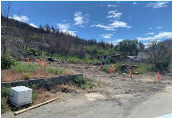
Figure 5 – Lot 665 Zone 6 Debris Removed
