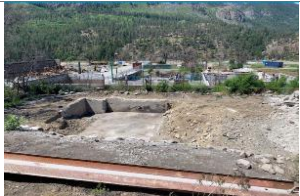
Figure 6 – Lot 420 Zone 5 Debris Removed
