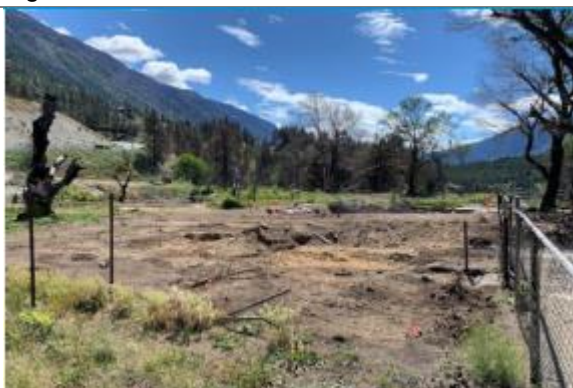
Figure 7 – Zone 1 Lot 47 and 57 Debris and Concrete Removed
