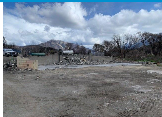
Figure 2 – Metal Debris Removal – 45 River Road
