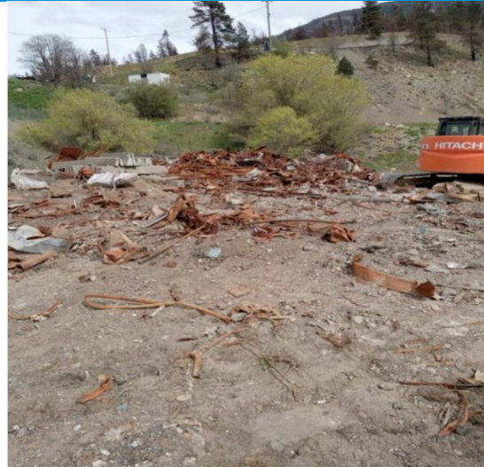
Figure 4 – Hobo Hollo - Debris removal on properties
