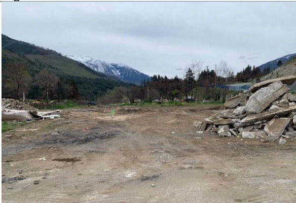
Figure 7 – Zone 1 Lot 84, 68, 58 debris and concrete removed
